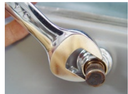
Fig 8: Above- Using the 3/4 open end wrench, tighten the chrome nut.
