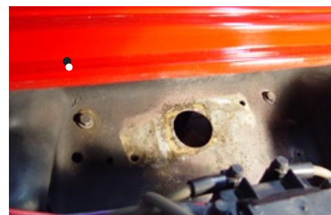
(Fig 08) See the pass side 1/4" bolt in the engine compartment.
